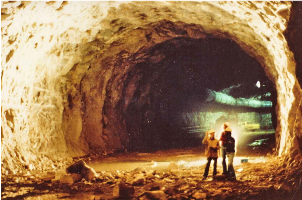
Figure 1: The 12 m span 8 m high top heading for the tailrace tunnel was constructed by full-face drill-and-blast and, because of the excellent quality of the massive gneiss, was largely unsupported.
